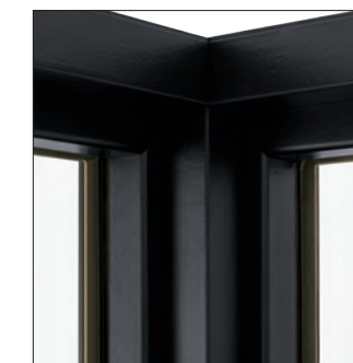
INTERIOR CLOSE UP
